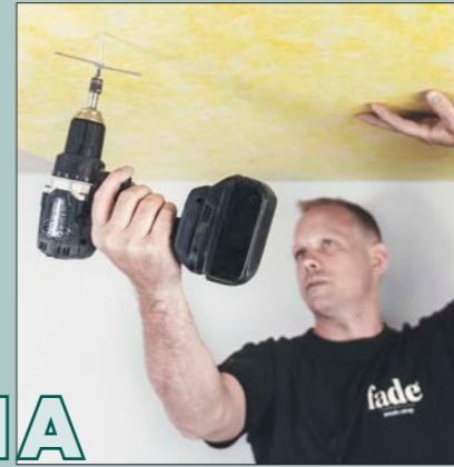
1A MECHANICAL INSTALLATION
