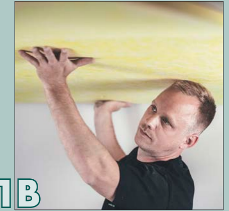
1B ADHESIVE INSTALLATION
