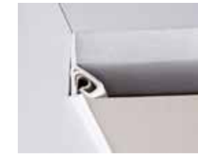
Clipso ceiling installation with PCW profile.
