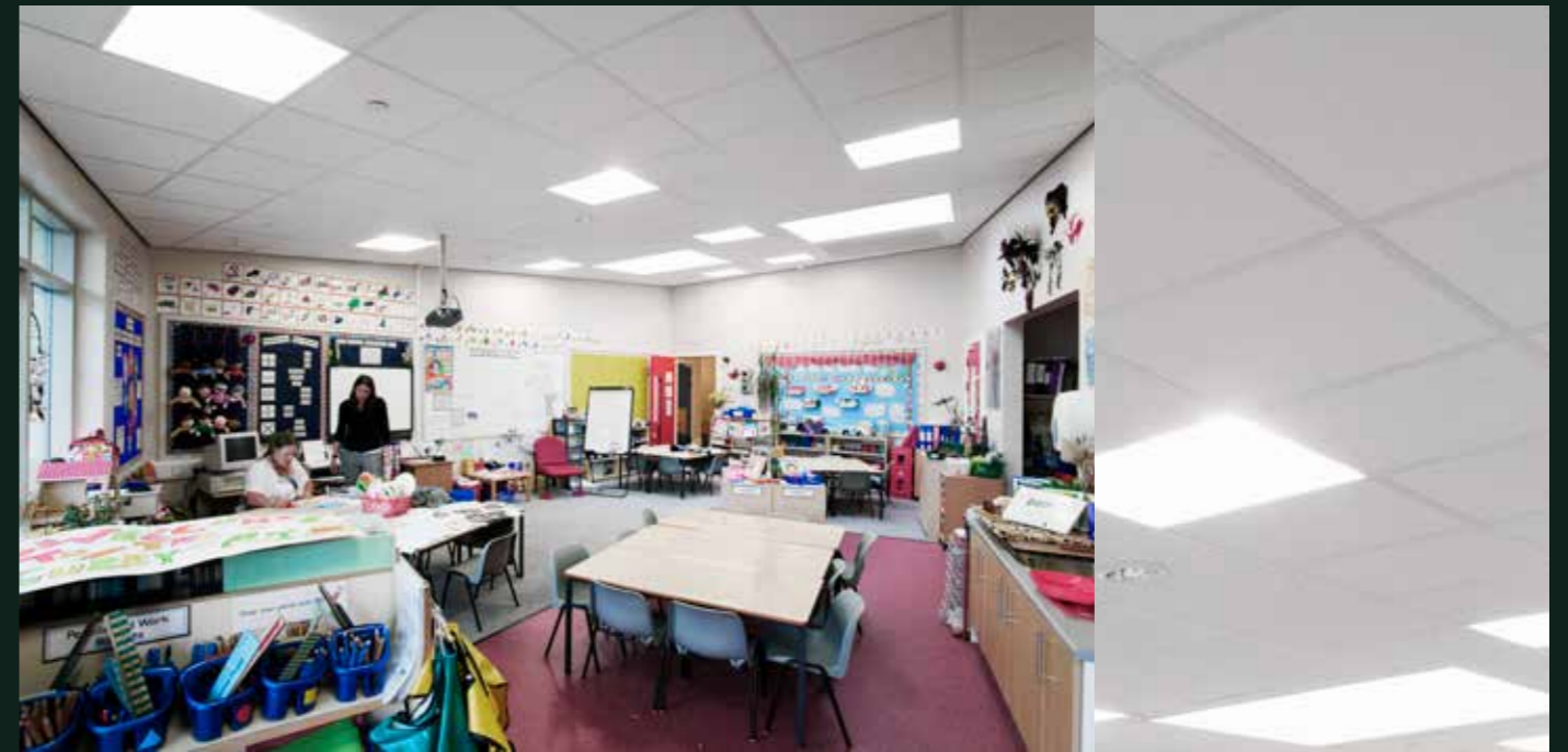
MASTER RIGID A Visible grid system with reinforced surface secured by clips but fully demountable tiles. Available in many formats.
