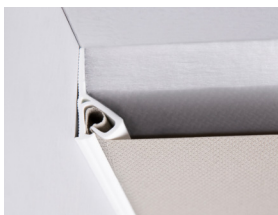
Clipso ceiling installation with PCW profile.
