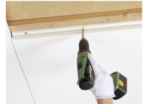
Master F is installed by screw fixing
