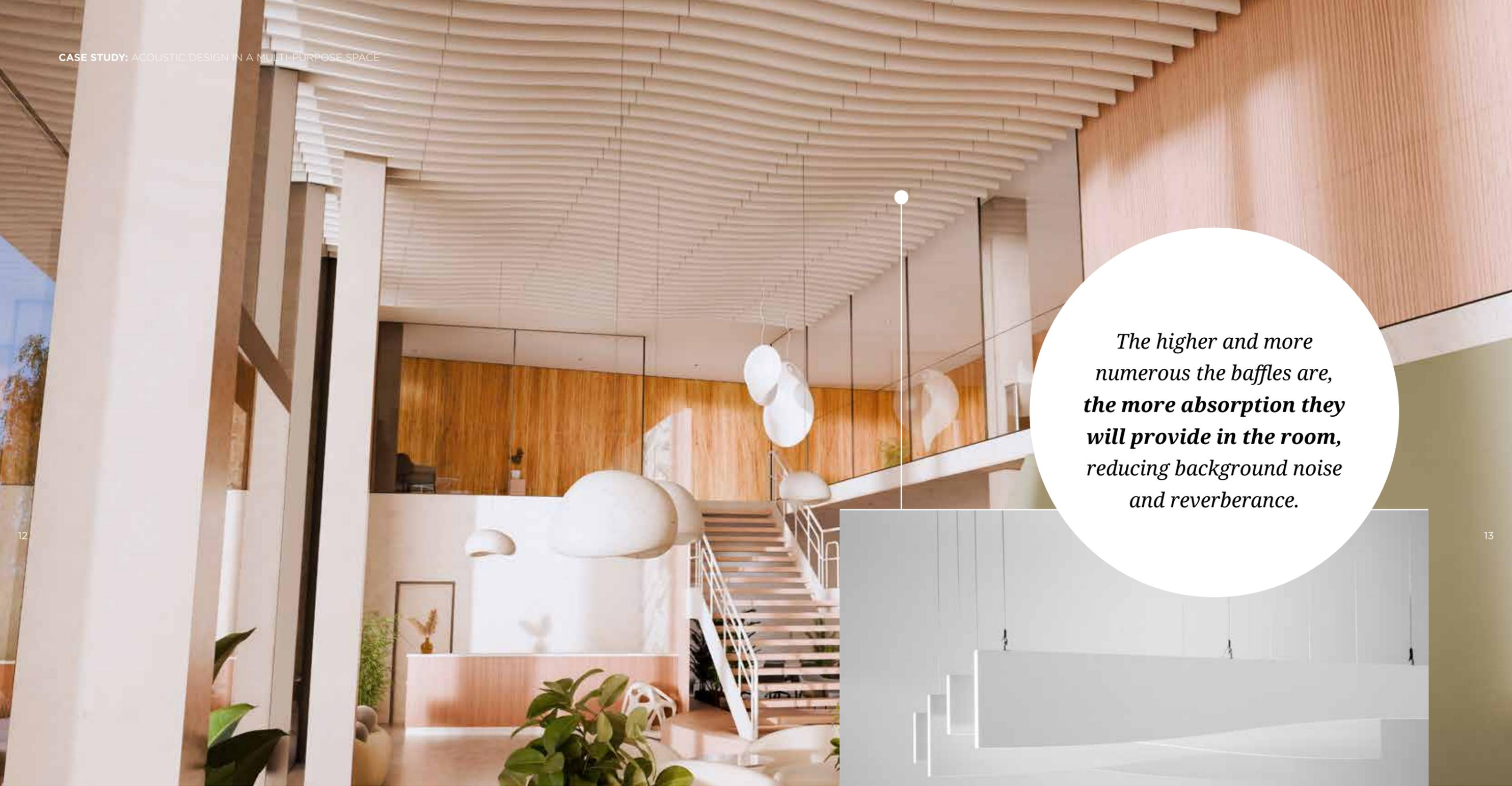
*The higher and more numerous the baffles are, the more absorption they will provide in the room, reducing background noise and reverberance.*
