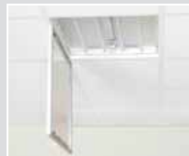
The frame is hinged to allow access to the luminaire
